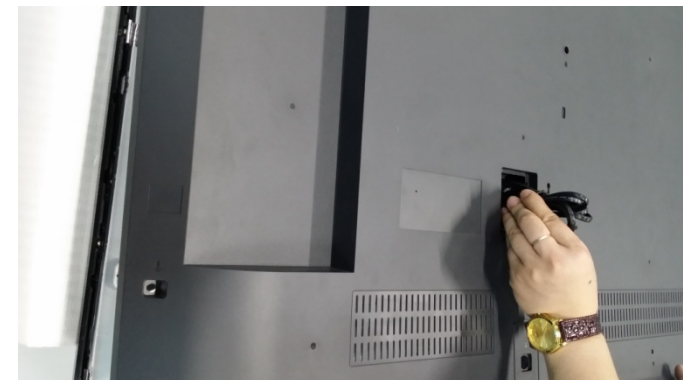
Insert the AC cord through the rear cover hole.
